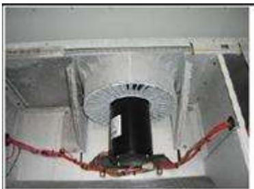
Analyses by Carrier Transicold environmental specialists have identified the white powder as consisting predominantly of aluminum oxide. Aluminum oxide is a coarse crystalline deposit most likely the result of surface corrosion on the aluminum parts within the container. If left untreated over time, it may build up in thickness and eventually flake as a light-weight white powder.
