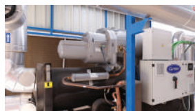
30XWH water/water koelmachines
