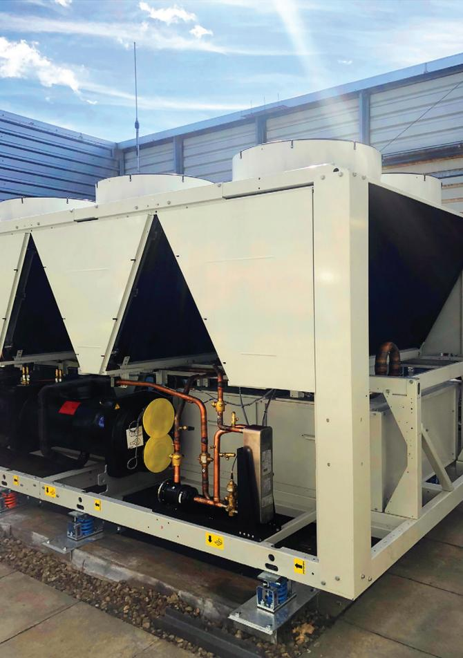
The first UK installation of Carrier's new ultra-low Global Warming Potential (GWP) AquaForce® 30XAV chiller operating on the company's PUREtec® HFO R-1234ze refrigerant has been completed at Gatwick Airport Ltd. Selected as a replacement for an ageing air-cooled screw chiller, the project is part of a major upgrade at Jubilee House, the administrative offices of Gatwick Airport Ltd.
