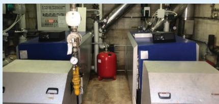
Before: boiler room
