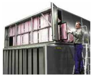
Filter row can be completely pulled out in one move
