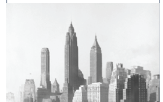
Carrier announced that the four biggest and most modern post-war skyscrapers in New York city would be air-conditioned from top to bottom by Carrier's Conduit Weather Master System.
