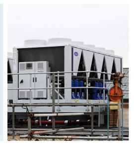
Options included enhanced acoustic attenuation to further reduce noise, and Enviroshield® condenser coil protection, with comes with a three-year warranty.
