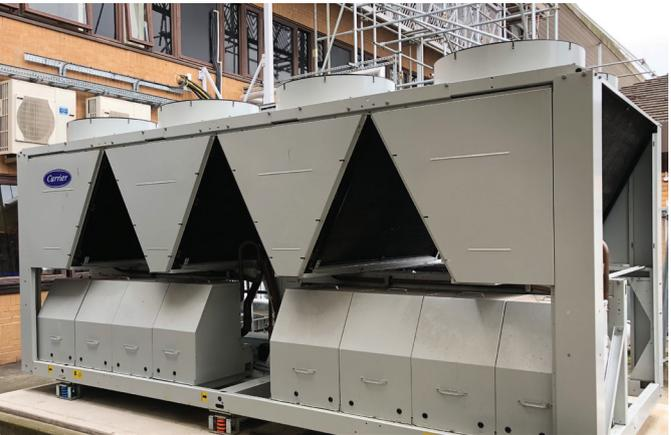
Carrier has supplied a high-performance Aquasnap® air-cooled chiller equipped with Super Enviro-Shield® condenser protection to Weston General Hospital. The chiller, installed by RTS Engineering Somerset Ltd, features Carrier's Super Enviro-Shield condenser coating, an extremely durable and flexible epoxy coating applied over all coil surfaces to completely isolate the metal and protect the all-aluminum heat exchangers from corrosion in the coastal climate.
