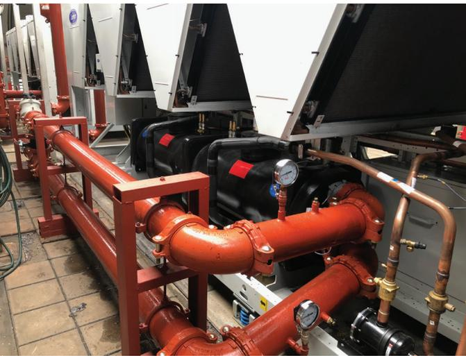
Two high performance Carrier air-cooled chillers with a combined cooling capacity of 1.17MW have been installed at The Royal Exchange in the City of London as part of a major refurbishment of premium office space in the iconic building.
