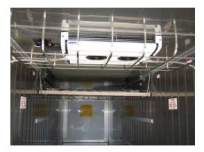
Refrigerant piping and wiring harness are mounted in box ceiling recess to guard against damage.
